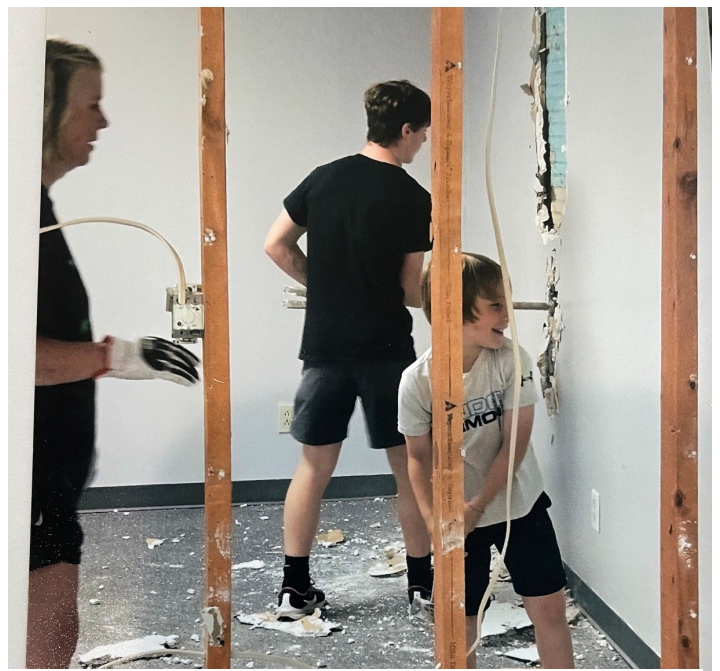
All ages helping with the renovation of Scarbro First Baptist Church.
