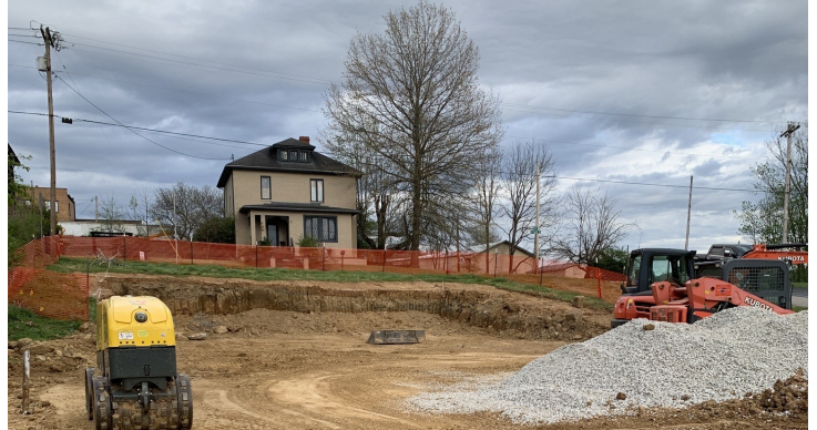
Construction begins for Harrisville Baptists' multipurpose building.
