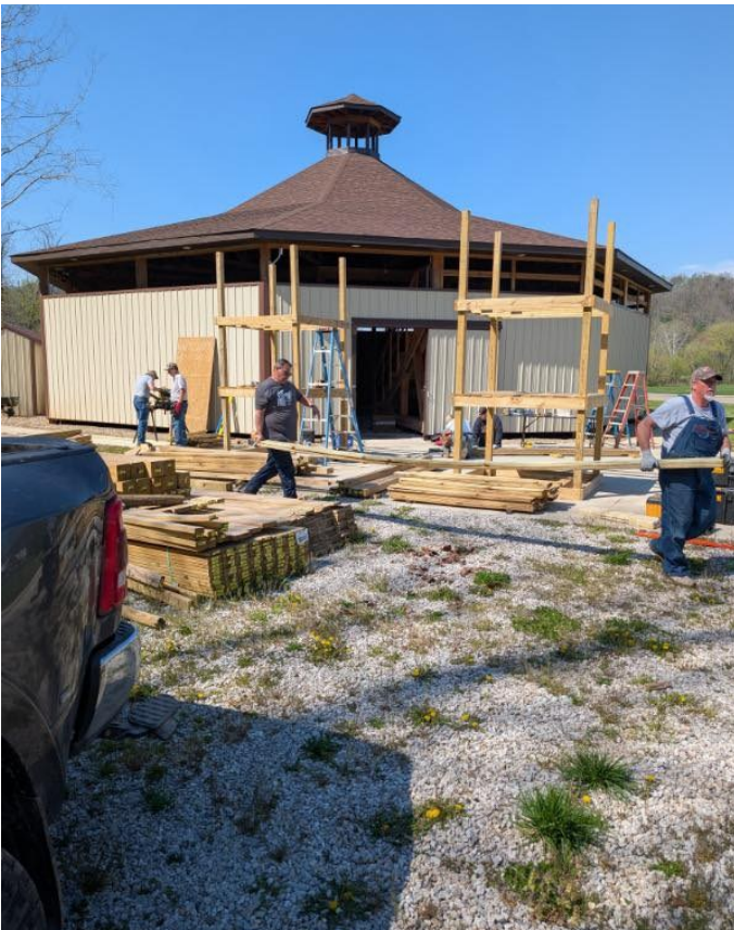
Beginning construction of the new playground at Parchment Valley.
