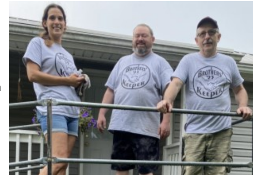
One BK team installed a handicap ramp for a homeowner's porch.
