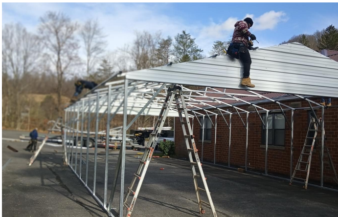
Construction of the outdoor pavilion at Flemington Baptist Church.
