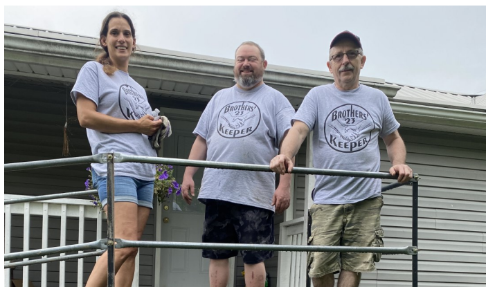
One of our BK teams installed a ramp on a homeowner's porch.
