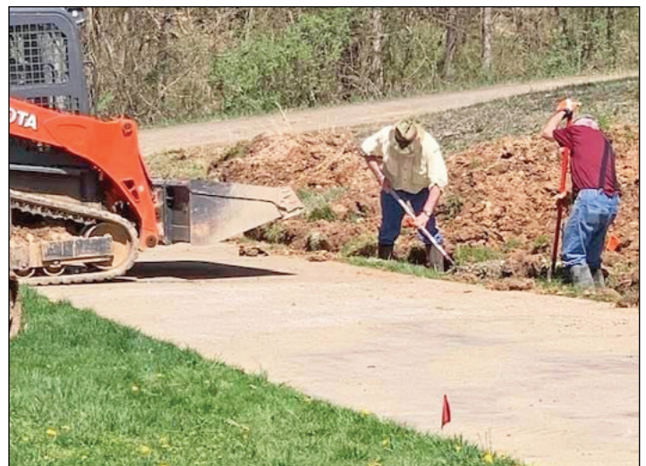
Tom Dale and Terry Mayfield working around the Mission House.
