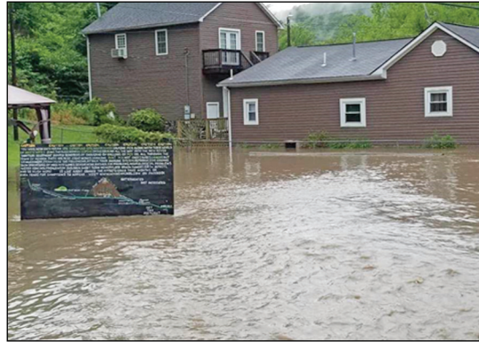
The recent rising flood waters in Fayette County
