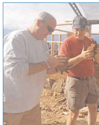
(l to r) Greg O'Neal and Jim Anderson form cobs for the walls of the home.
