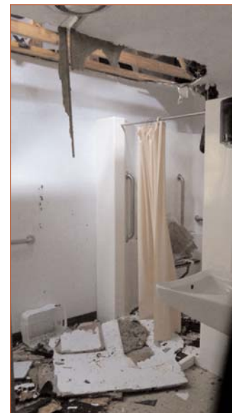
The results of a tree falling through the roof of the Milam-Hopewell cabin.
