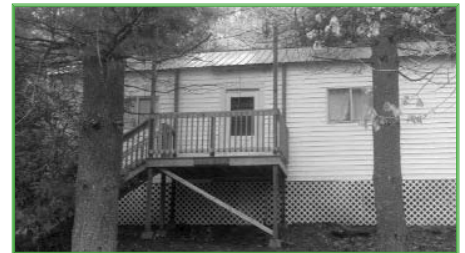
A porch has been added to the Broad Run (above) Association cabin.
